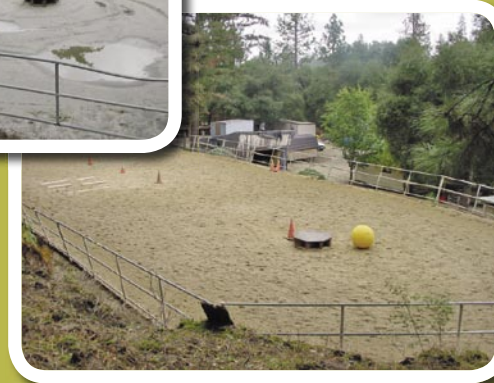
» AFTER: Proper drainage significantly reduced pooling and sediment runoff
