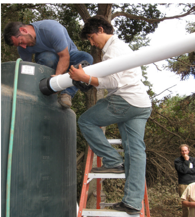
A cistern captures runoff from the paddock roof and uses it for watering the horses and arena dust control
